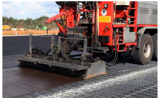
Figure 1. The concept of the Mesh Track® implementation in a road structure
