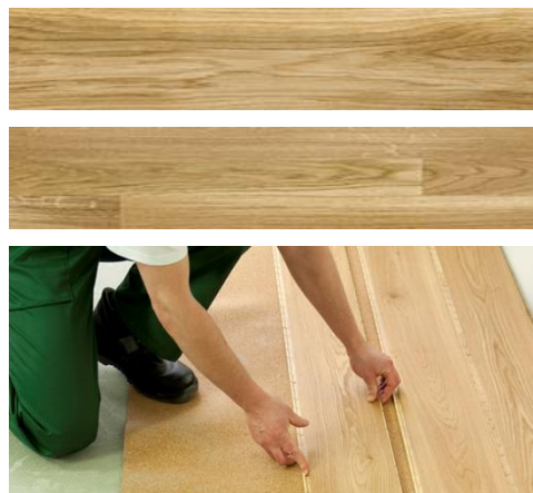
Fig. 3. The view of 3-layer wooden floorboard during installation
