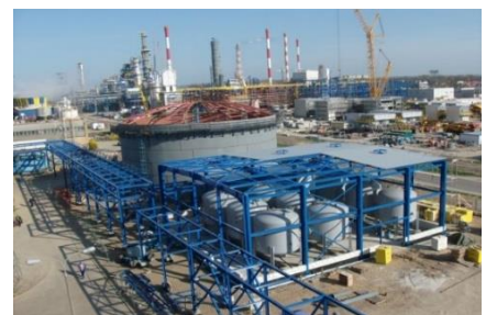
Fig. 5. Sewage treatment plant of Lotos group (Poland)
