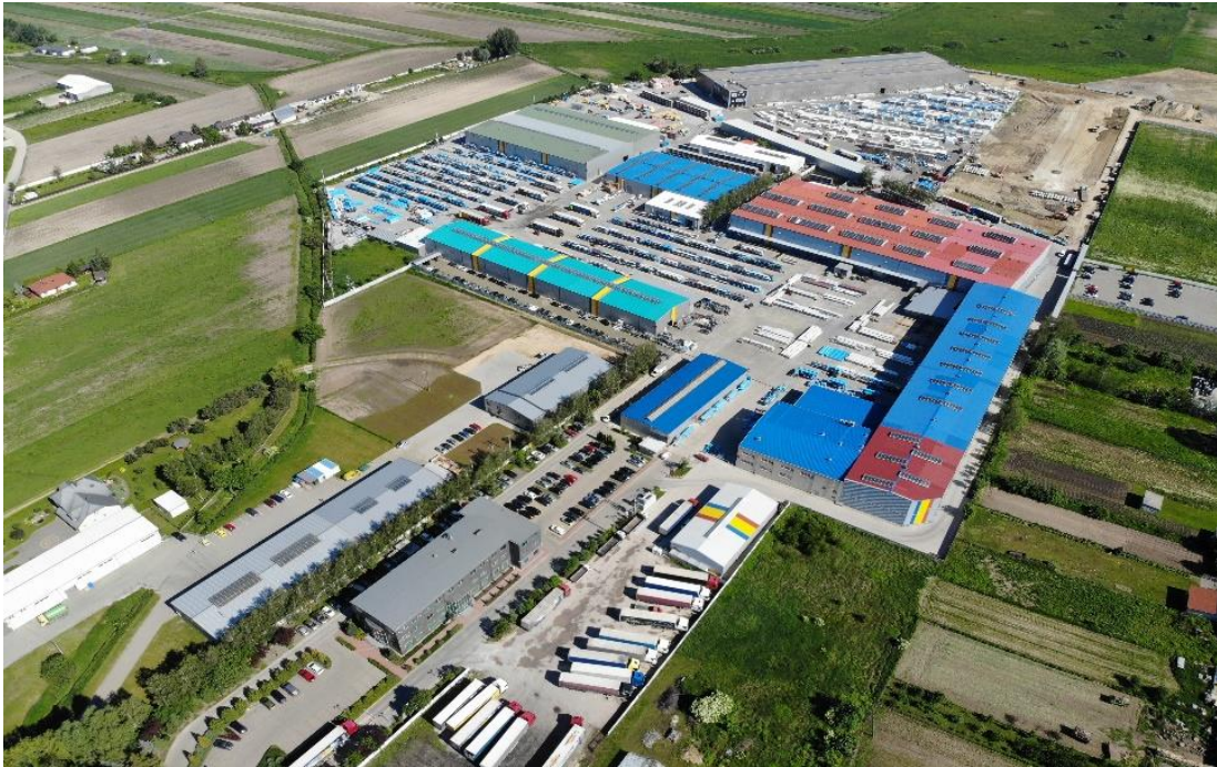
Fig. 1. A view of the Pruszyński Sp. z o.o. production hall in Sokolów (Poland).
