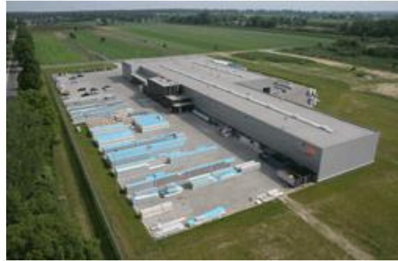
Fig. 1. The view of ArcelorMittal Construction Sp. z o.o. plant in Rawa Mazowiecka.
