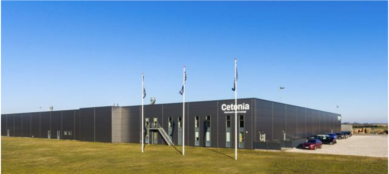
Fig. 1. Cetonia A/S manufacturing plant located in Bjerringbro, Denmark.
