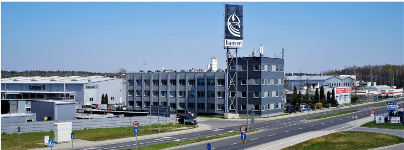
Fig. 1. Hansen Polska manufacturing plant located in Głogów Małopolski, Poland.
