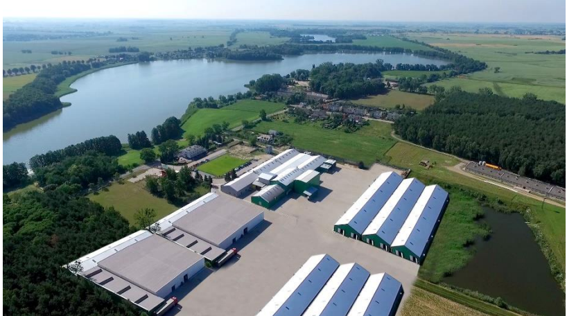
Figure 1 Fair Packaging production plant in Buszewo, Poland
