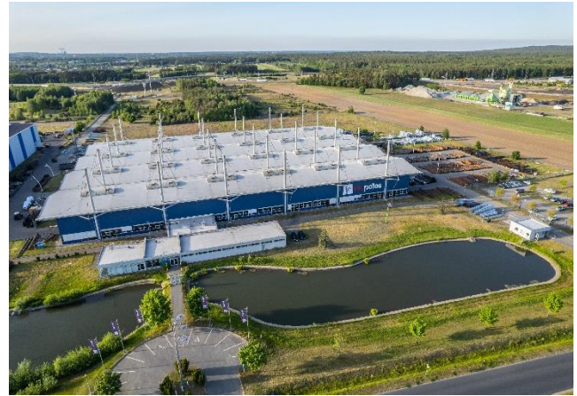
Fig. 1. The view of the company headquarters of Tecpoles Sp. z o.o. in Kragola.
