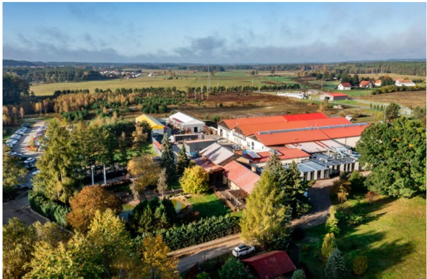
Fig. 1 The main manufacturing plant in Wilimowo, Poland
