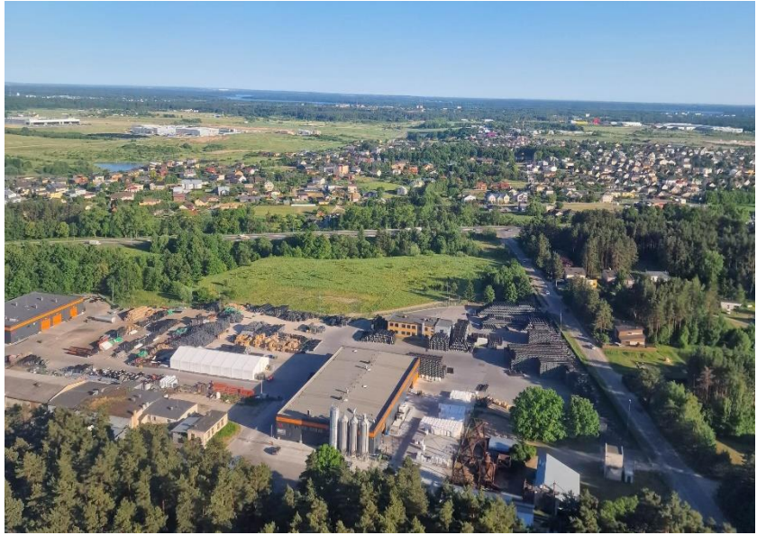
Fig. 1. A view of UAB ViaCon Baltic Pipe steel manufacturing plant (Margava, Lithuania)
