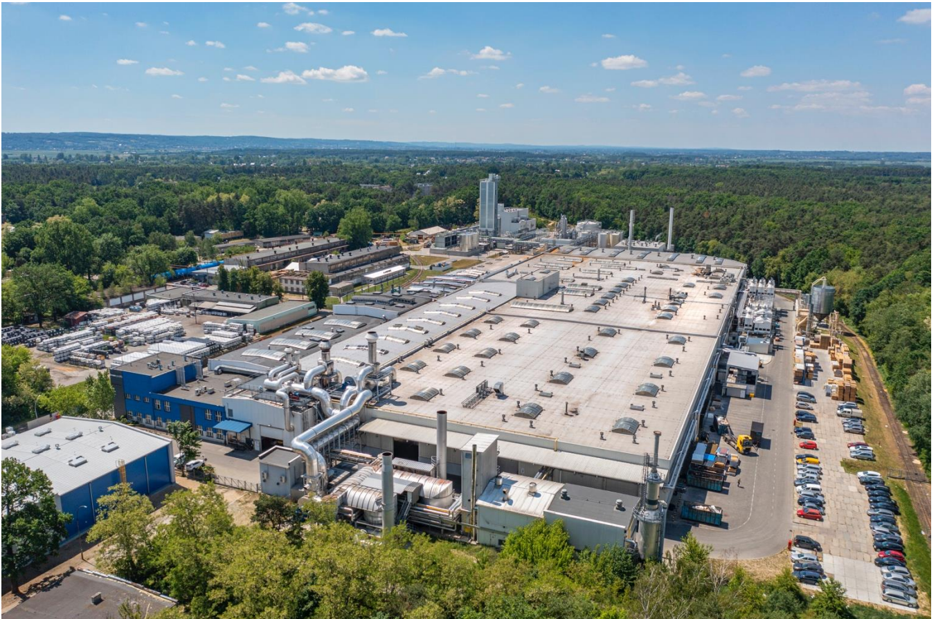
Fig. 1. A view of Kronospan HPL Sp. z o. o. in Pustków (Poland).
