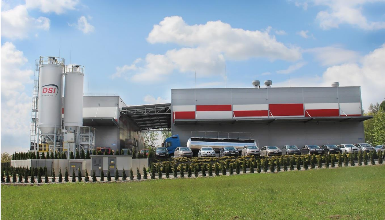
Fig. 1. A view of the DSI Underground Chemicals sp. z o.o. production plant located in Mikołów (Poland)
