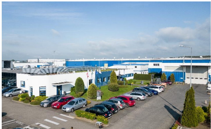
Fig. 1. A view of manufacturing plant
