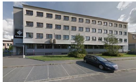
Fig. 1. The view of Track Tec KolTram Sp. z o.o. in Zawadzkie.
