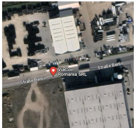
Fig. 1. A view of VIACON ROMANIA SRL manufacturing plant (Prejmer, Brașov)
