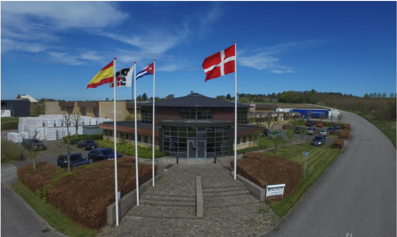
Figure 1: A view of the DC-System Insulation A/S production plant located in Aars (Denmark).
