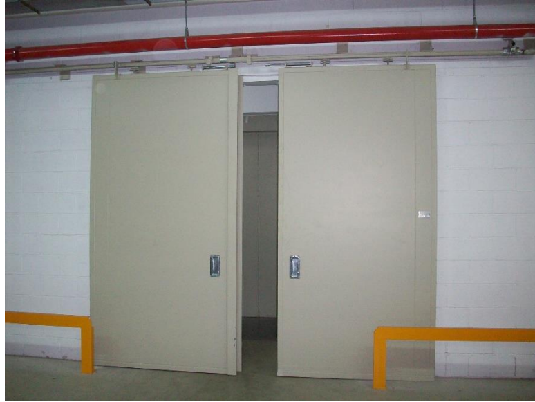
Fig. 2. Sliding fire gates produced by NGR Technologie.
