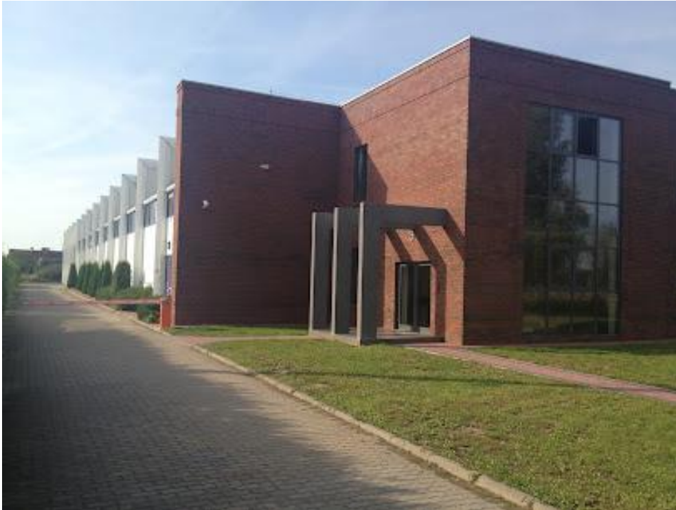
Fig. 1 A view of NGR Technologie Sp. z o.o. production plant located in Grodzisk Wielkopolski (Poland).
