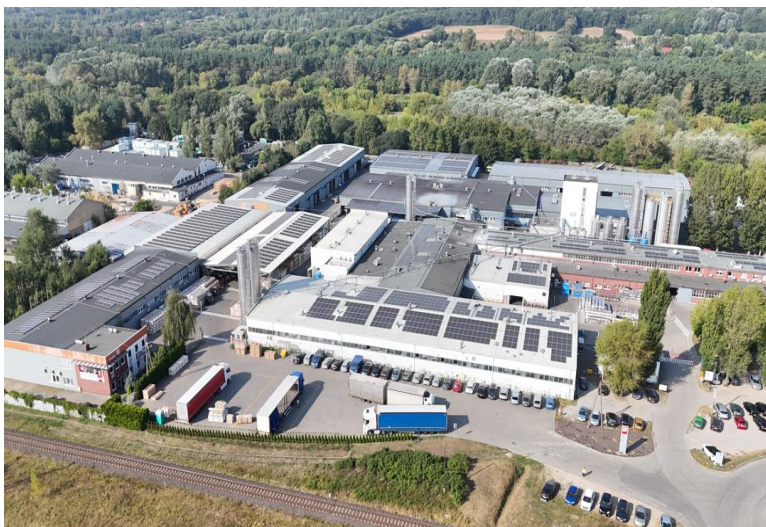
Figure 1 A view of production plant located in Czerwonak (Poland).
