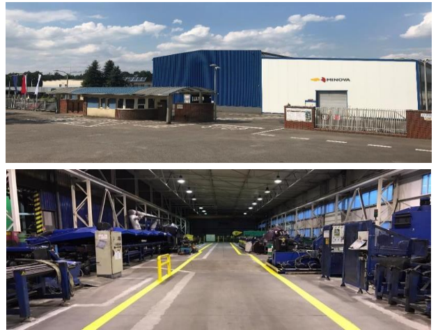
Fig. 1. Manufacturing Plant in Golce.
