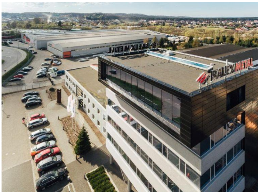
Figure 1 A view of Balex Metal production plant located in Bolszewo (Poland).
