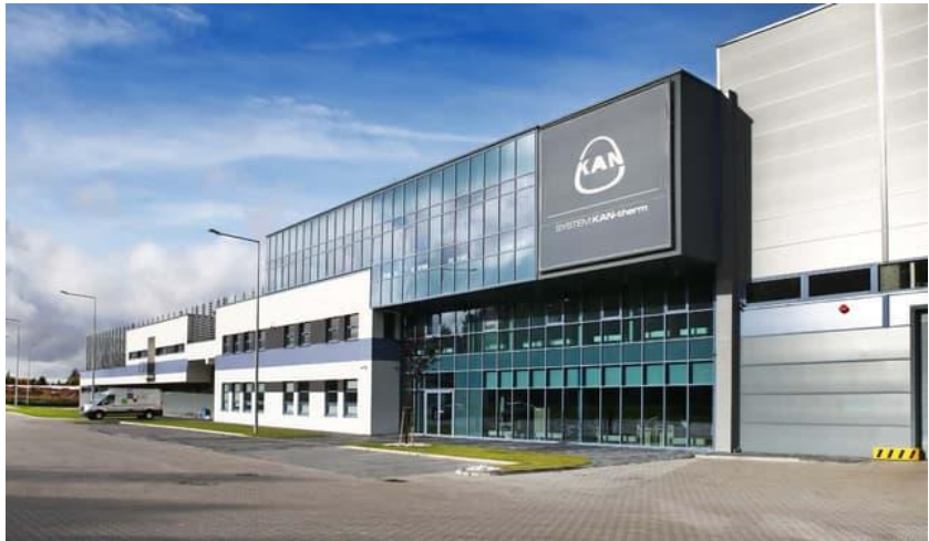
Figure 1 The view of KAN Sp. z o.o. manufacturing plant located in Kleosin
